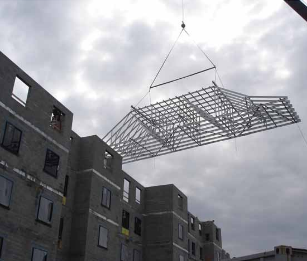
Staybridge Suites - Glen Mills, PA
